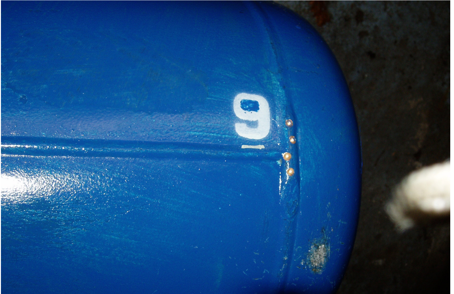
PHOTO 9: WELD CAP PITTING
