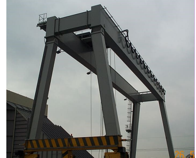
The overhead crane
